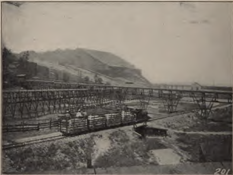
PLANT TRANSPORTATION OF DYNAMITE.
