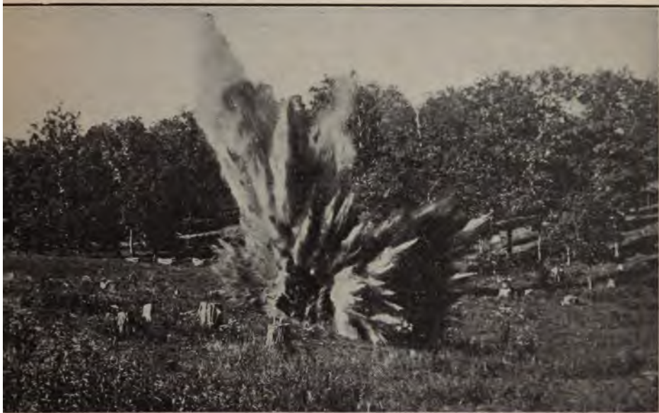
BLASTING A STUMP—"A TOUGH CUSTOMER EASILY REMOVED."
