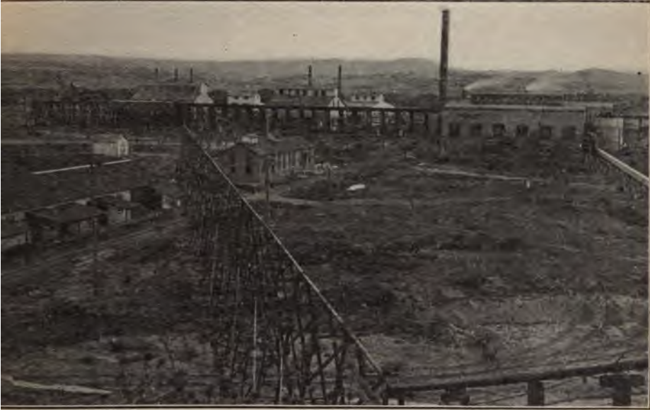
POWER HOUSE AND ACID PLANT, LOUVIERS, COLORADO.
