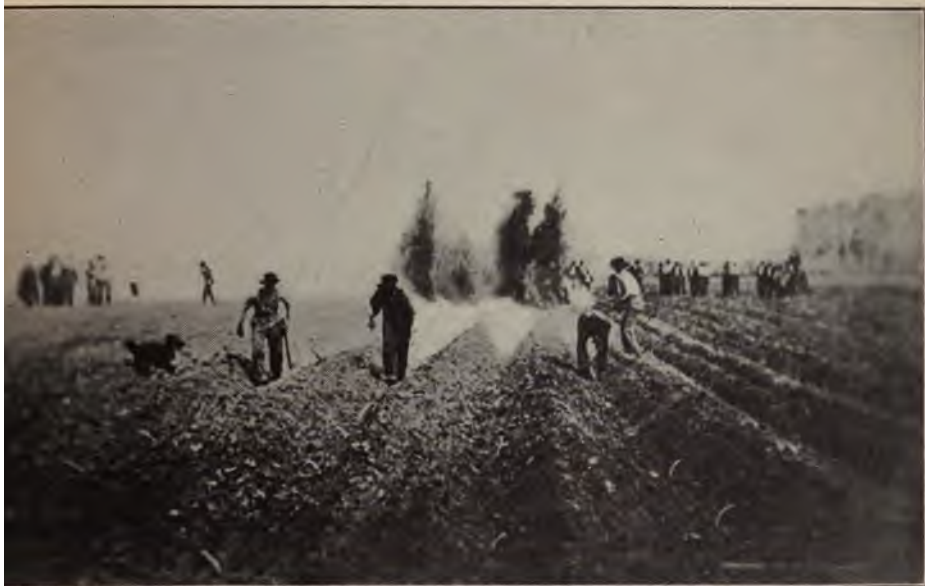
SUBSOILING WITH DYNAMITE—LIGHTING THE FUSE.
