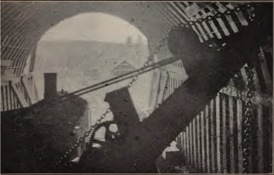
NORTHERN PACIFIC TUNNEL, KELSO, WASH.
