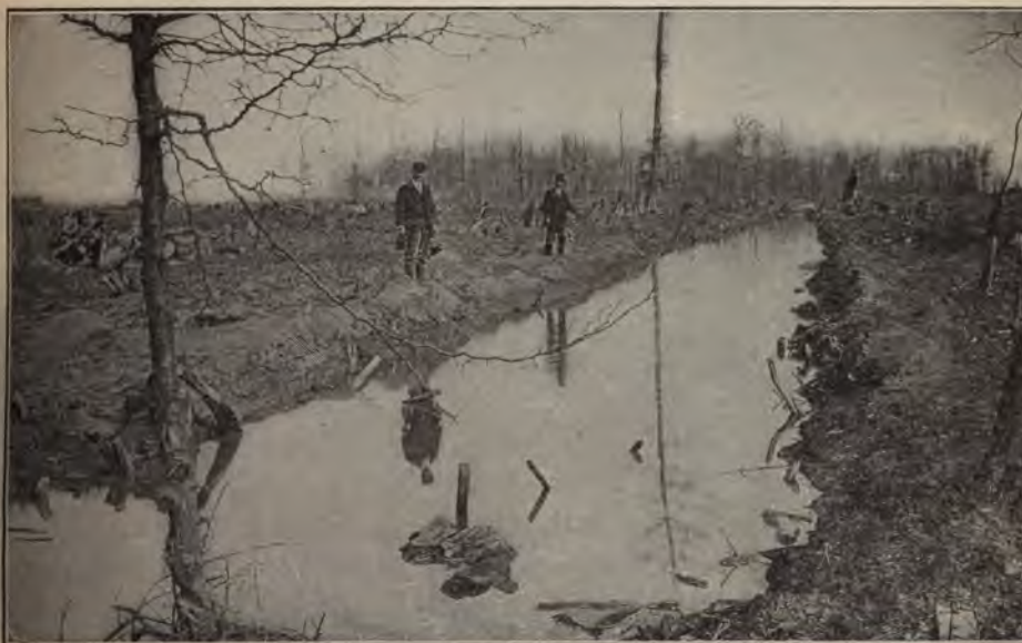
BLASTING A DITCH—AFTER THE WATER HAS BEEN LET IN.
