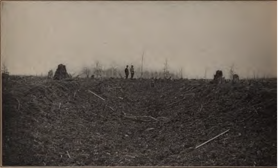
BLASTING A DITCH—AFTER THE BLAST.
